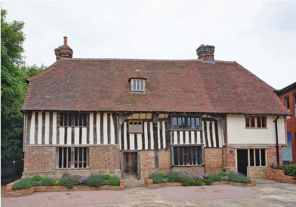
Fig. 2. Bridge Cottage today.
