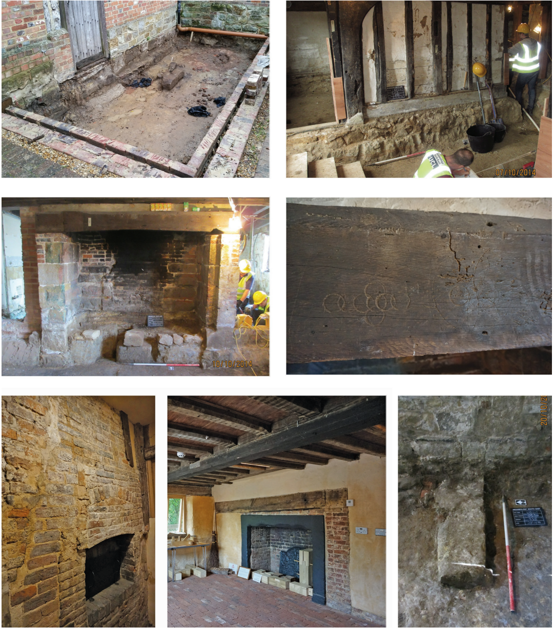
Fig. 20. Photos, Period 4. Top left: yard area with G32 in background; top right: G24 facing south; centre left: G26 fireplace looking north; centre right: witch marks on G26 lintel; bottom left: oven inserted into rear of kitchen fireplace; bottom centre: kitchen fireplace; bottom right: G28 buttress.
