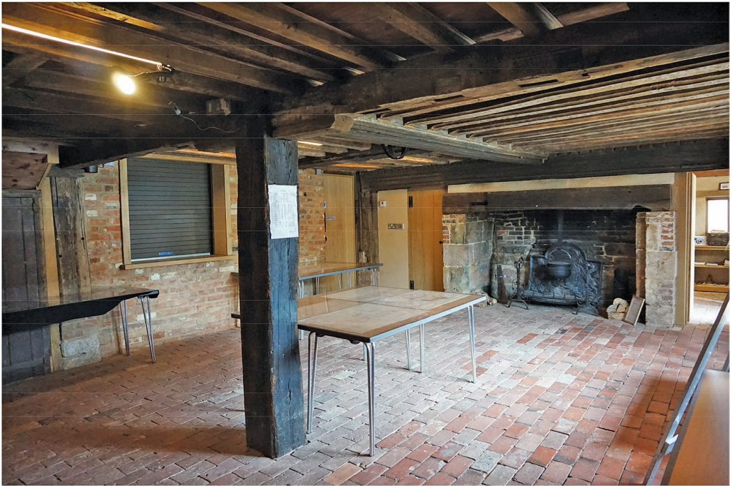
Fig. 15. Interior of Bridge Cottage during Period 2. Top: reconstruction looking towards the dais partition and high table (courtesy of David Martin); bottom: following restoration (with the floor and chimney inserted).
