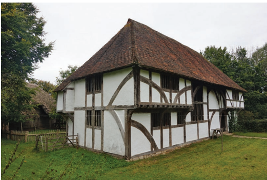
Fig. 16. The projecting garderobe (rear left corner) as reconstructed at Bayleaf, from Chiddingstone, Kent, now at the Weald and Downland Living Museum.
